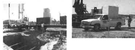
Installing a below-grade Optical NOC (below)
