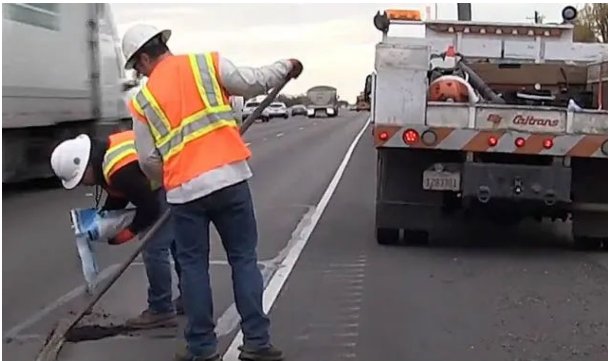
A Caltrans crew repairing a highway. Courtesy Caltrans
